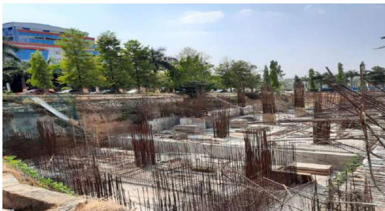
Photo: Ongoing Construction Works
