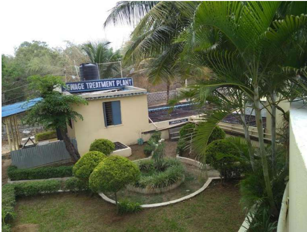
Photo : Sewage Treatment Plant (250 KLD)
