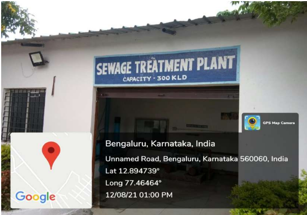
Photo: Sewage Treatment Plant
